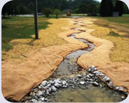
Wilson Park stream restoration project under construction in Lenoir, NC.
